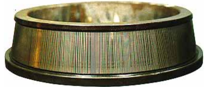
Figure 17: Fluting in the inner ring raceway of a tapered roller bearing was caused by the constant passage of current
